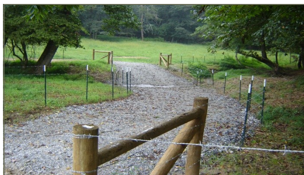
Stream Crossing with Buffer Fence
